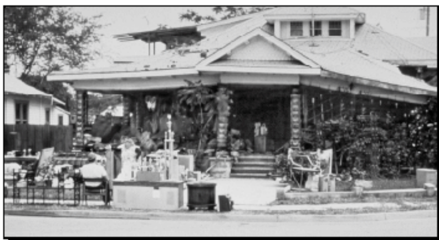
Damage from magnitude 6.7 earthquake
