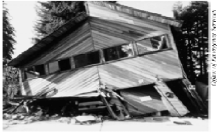
Figure 29 - This mountain home was built over a garage, and its walls were not strong enough to withstand an earthquake.
