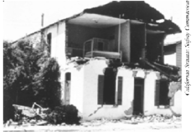
Figure 25 - The plaster-covered brick walls of this building collapsed during a recent earthquake.
