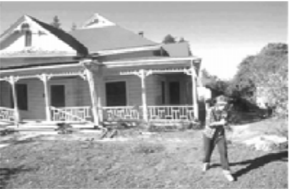
Figure 2 - Loma Prieta Earthquake, Oct. 17, 1989 Home moved off of its foundation and was considered a total loss.
