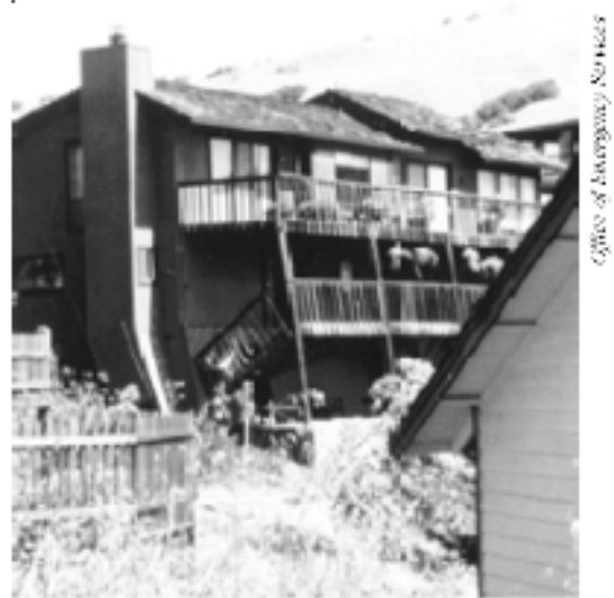
Figure 22 - This hillside home was built on an unbraced tall wall that failed.
