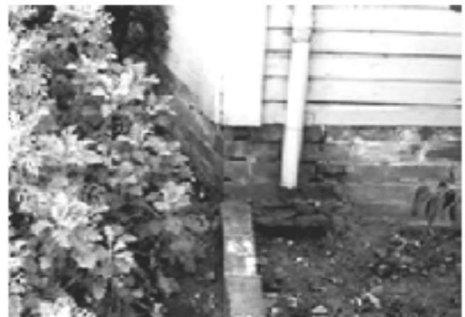
Figure 20 - Note the bricks exposed in this unreinforced masonry foundation.
