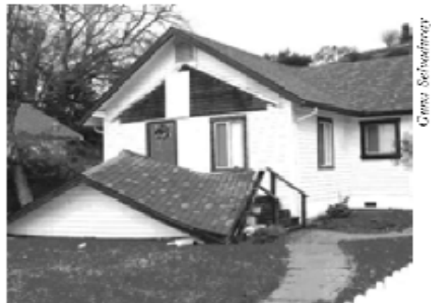
Figure 6 - San Simeon Earthquake, Dec. 22, 2003 The collapsed porch was not adequately attached to this single family residence.
