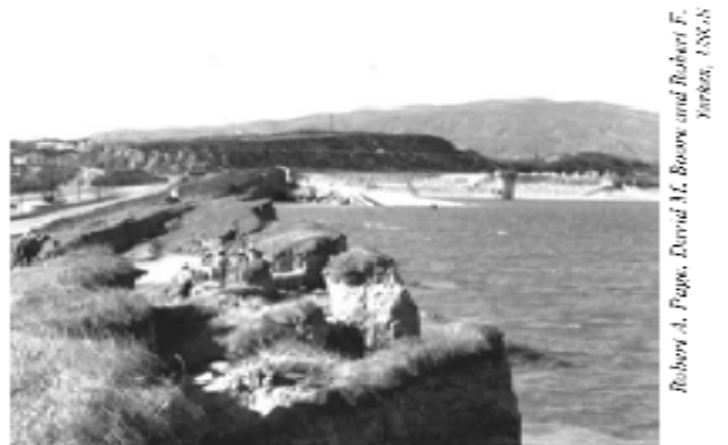
Figure 41 - Lower San Fernando Dam that was badly damaged by the 1971 San Fernando Earthquake.
