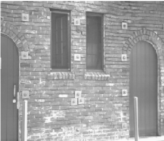
Figure 28 - Bolting of unreinforced masonry wall to steel frame on the inside.
