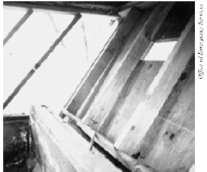
Figure 23 - This photograph shows an interior detail of a home similar to the one above, showing substantial damage to a building with an unbraced tall wall.
