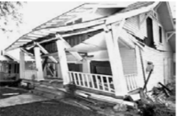
Figure 3 - Northridge Earthquake, Jan. 17, 1994 Single family residence damaged due to failure of multiple elements.
